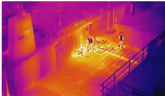
Photo: City of Bergen Fire Department
